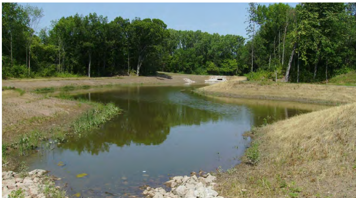
Figure 12.4 - Small constructed wetland for stormwater detention and water quality improvement (image courtesy of uncs.edu)
