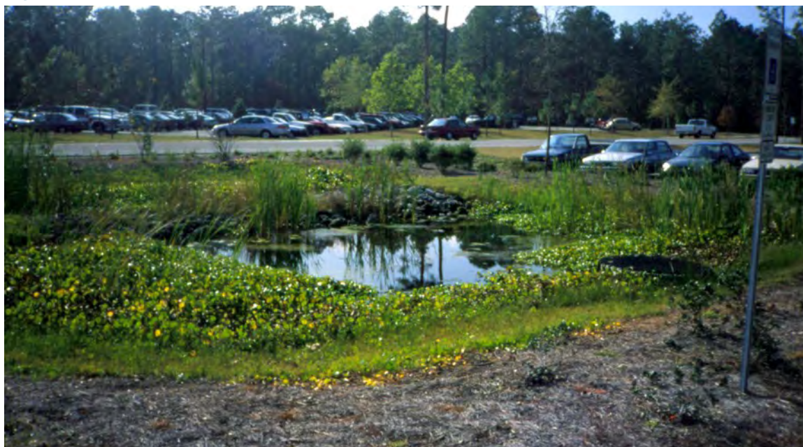
Figure 12.4 - Small constructed wetland for stormwater detention and water quality improvement (image courtesy of uncs.edu)
